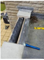
The cavity tray provision is the third and final line of defence in parapet construction. The failures range from poor cavity tray joint detailing, inadequate support and incorrect or lack of adequate provision for removal of trapped from the cavity.
