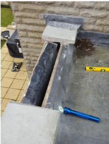
Failures in the horizontal DPC are common place. In the image to the left, we can identify a DPC of incorrect width, a lack of support to the DPC as it crosses the cavity and a lack of sealed joints in the DPC. The image to right shows a complete omission of the DPC, which has compounded the cavity tray issue (described below).
