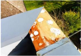
Image top left represents a situation where the DPC and DPC support has been omitted. As a result mortar bedding is not present and the copping has detached. Image top right represents a situation where the DPC has been omitted and the capping has been attached using mastic. Adhesion has failed and the lack of mechanical fixing has resulted in detachment and water ingress.
